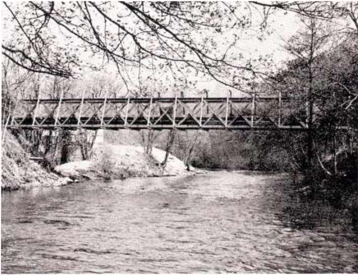
Strengthened Pipe Bridge
