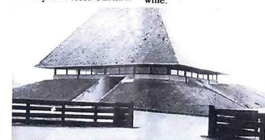
● The main pump-house at Ompton, housing one borehole, two booster pumps and all the control gear. Passing motorists have been seen to pull up and stare at the three similar style 1960's pyramids.
